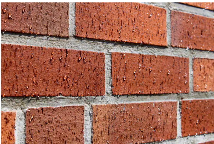
Fig.2 Impregnated facade. Water beads off and the building material is dry.
