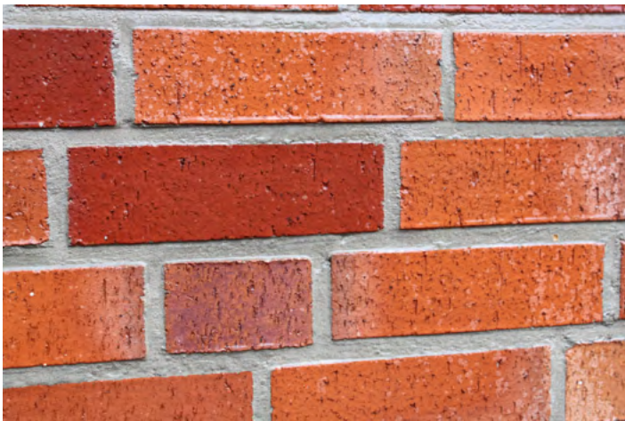
Fig.1 Untreated facade. Water is absorbed by the building material.
